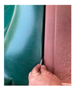
The loose rubber measured between 2" and 4" and non-compliant. A minimum of 6" is recommended. CPSC 2.4.2.2. and ASTM F1292
