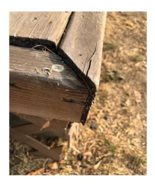
The three items in the photos fail the eye socket gauge and are protrusions.
