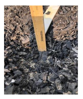
The ground is recessed with elevated concrete where a child could trip. CPSC 3.6. Fill in low areas.
